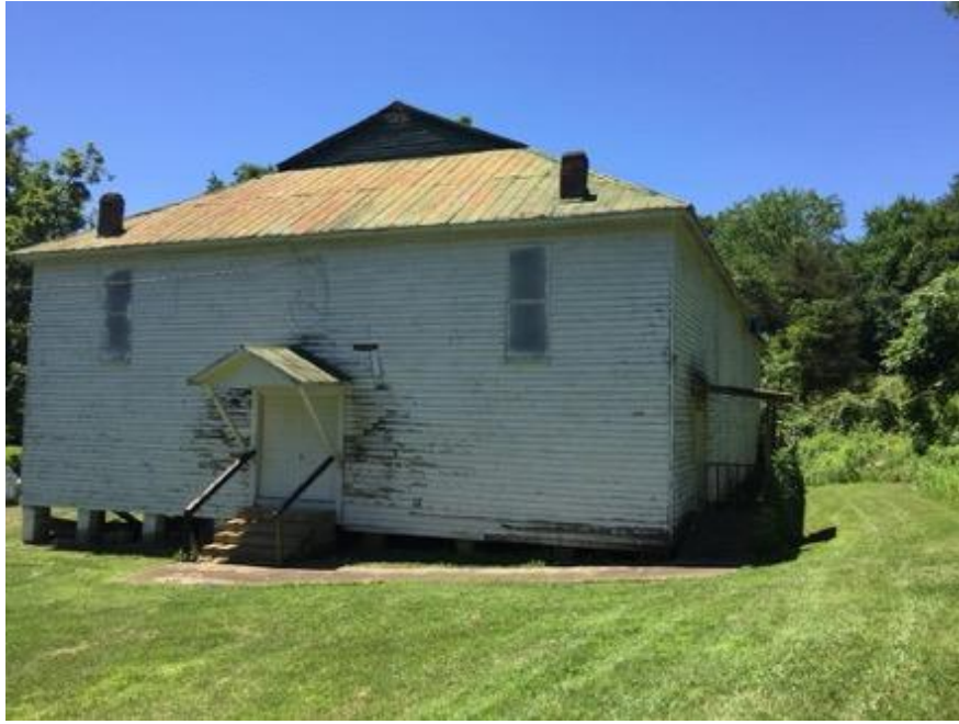
Figure 10-11: The Shady Grove School and Gymnasium following restoration efforts. Photo taken by author, Summer 2019.
