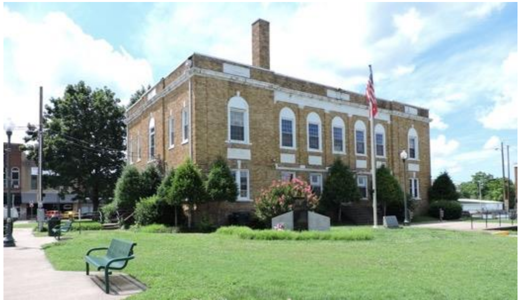
Figure 1: Centerville historic 1925 courthouse. Photo taken by author, Summer 2019
