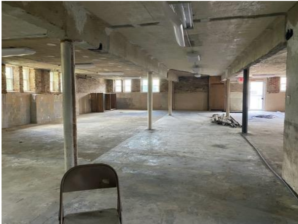
Figure 20: Current state of the basement of Courthouse, Image taken by author, Spring 2020
