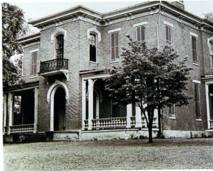
Figure 3: Pinewood Mansion. Courtesy of the Tennessee State Library & Archives
