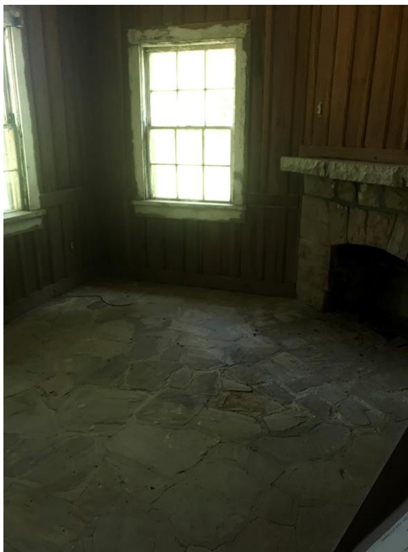
Fig. 5.13. Assistant Director's office featuring a sandstone floor and fireplace, 2020.
