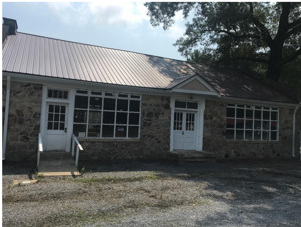
Fig. 5.9. Front of Commissary showing new roof and windows. Windows were returned to New Deal-era location, 2020.
