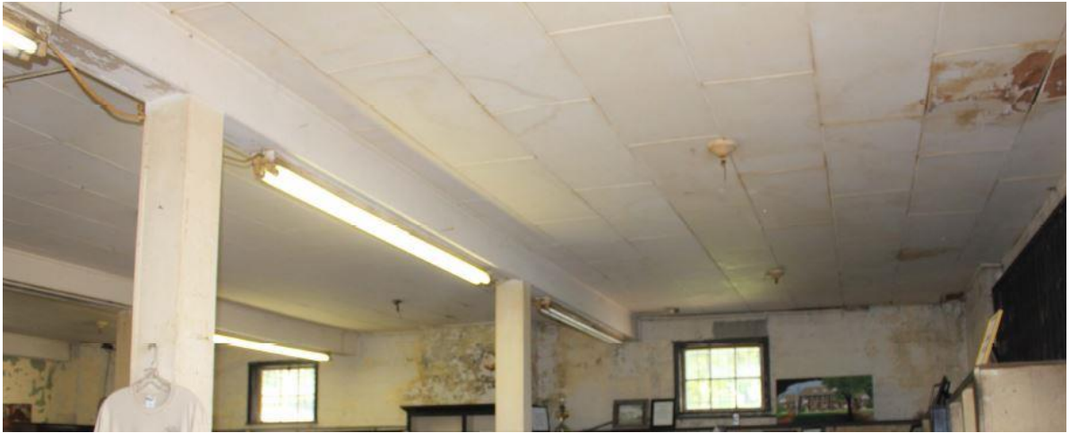
Fig. 5.4. Interior of Commissary ceiling and interior lighting, 2010.
