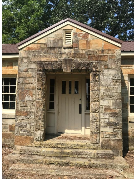
Fig. 5.11. Entrance to Administration Building, 2020.
