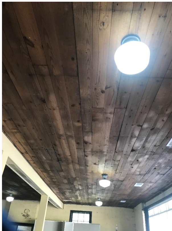
Fig. 5.5. New ceiling interior and historically appropriate lighting, 2020.
