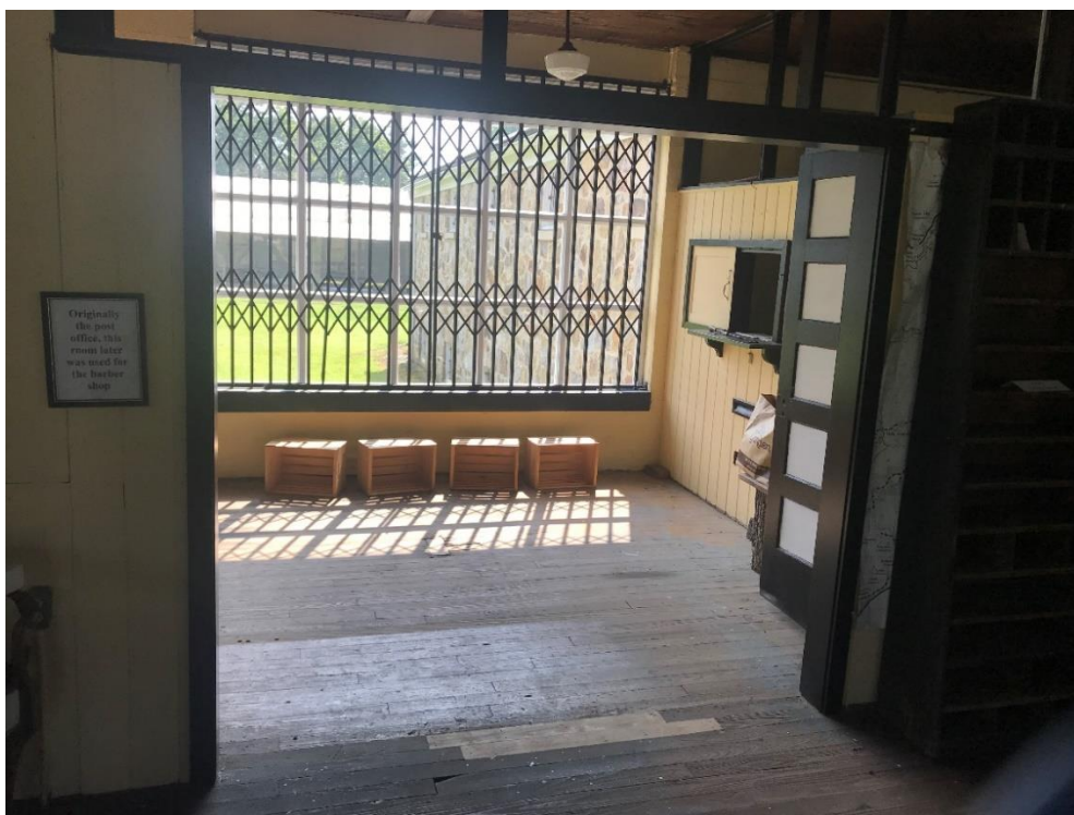
Fig. 5.7. Old doorway torn down and area opened, floorboards replaced, windows replaced; area now serves as gift shop and leads to new restrooms, August 2020.
