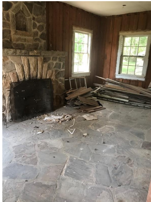
Fig. 5.16. Debris in former construction manager's office, 2020.
