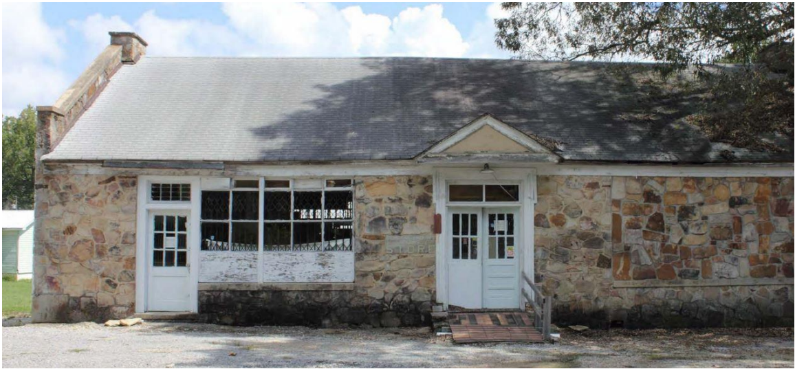
Fig. 5.8. Front of Commissary building, 2011.
