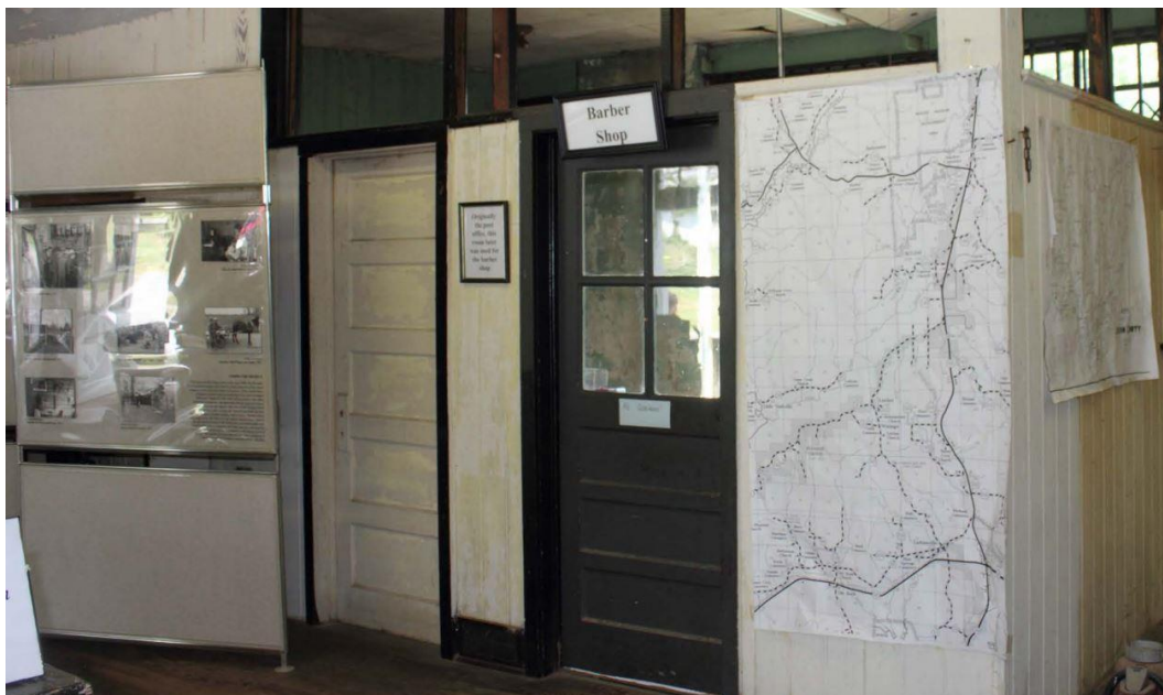
Fig. 5.6. Entrance to former barber shop area; closed off due to structural issues with floor and windows, 2011.
