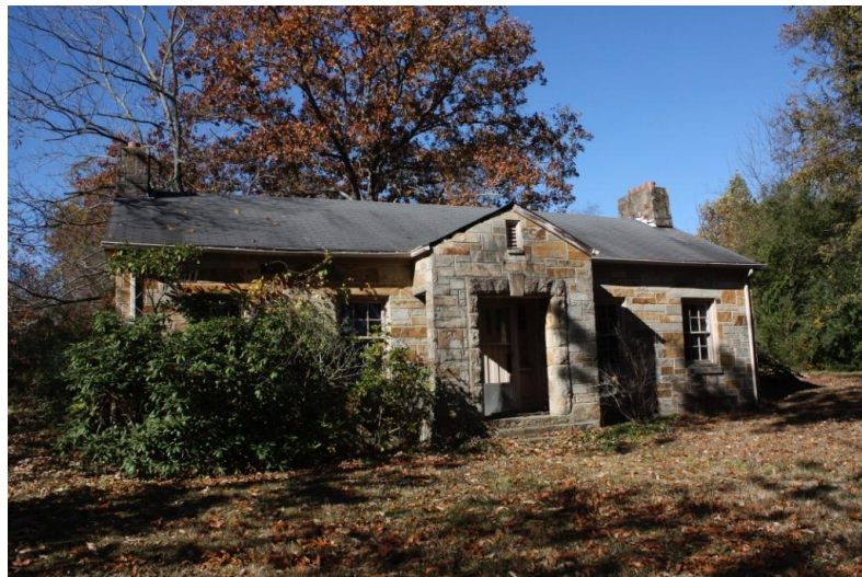
Fig. 5. 10. Exterior of Administration Building, prior to renovations, 2015.
