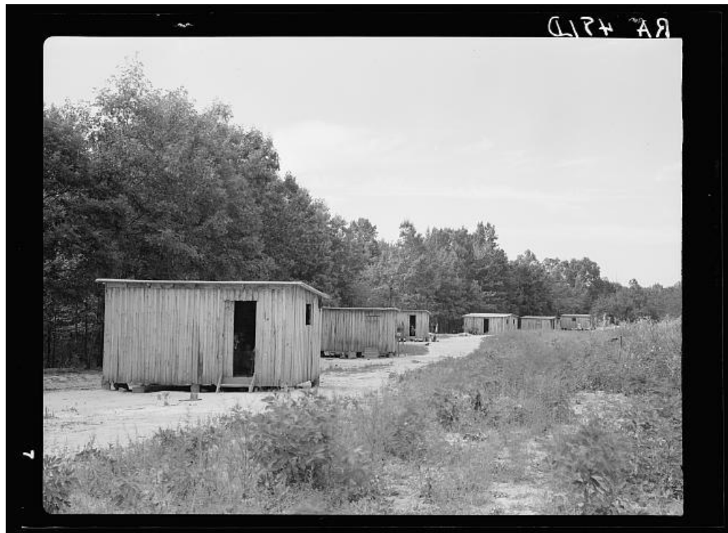
Fig. 4.1. Temporary shacks used by resettlement families while new homes are being constructed. Skyline Farms, Alabama, September 1935. 217
