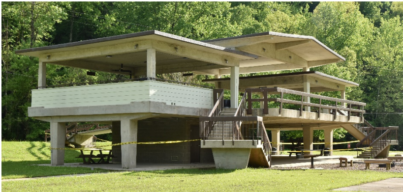
A pavilion at Rock Island State Park is blocked off with yellow caution tape in April 2020 for social distancing measures. (Photo by Madeline Quinby)
