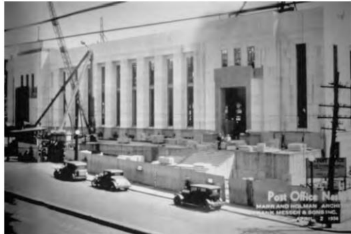
The Post Office on Broadway (now the Frist Center for the Visual Arts) under construction. (Photograph, April 2, 1934: Marr and Holman Collection, The Tennessee Historical Society, Tennessee State Library and Archives) Kreyling
