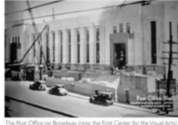
The First Office on Broadway. Once the First Center for the Visual Arts, under renovation. (Photograph April 1, 2014. Photo by Robert G. Anderson. The Tennessee Historical Society, Tennessee State Library and Archives) Kreyling
