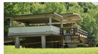
A pavilion at Rock Island State Park is blocked off with yellow caution tape in April 2020 for social distancing measures. (Photo by Madeline Quinby)
