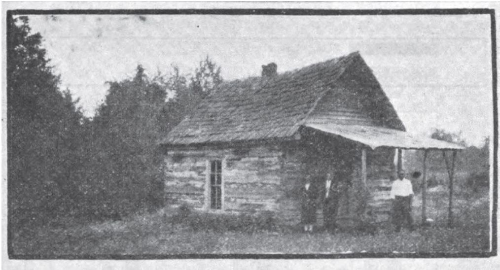
Image 10 - Rural Hill ME Church and School, pictured here around 1925, served the Duplex African American community from as early as the late 1860s, as a main classroom, until the around 1950, when it was still used as a classroom. A Study of Local School Units in Tennessee , 1937.
