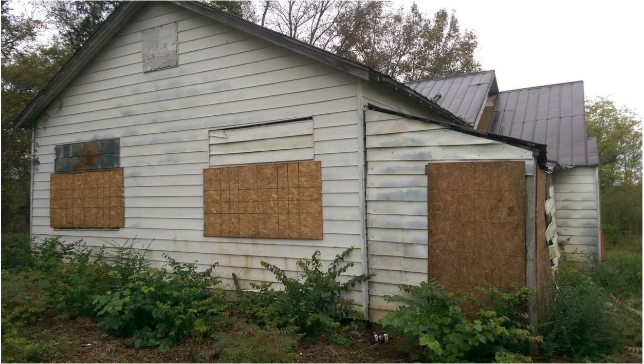
Image 54 – East elevation of Lee-Buckner School building, 2020
