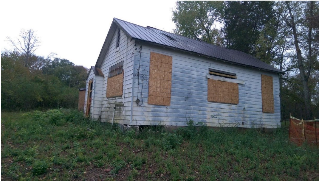
Image 55 – West elevation of Lee-Buckner School building, 2020.
