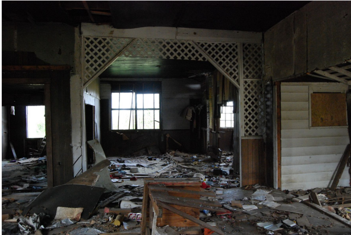
Interior of Lee Buckner School looking into original school room (March 2012).
