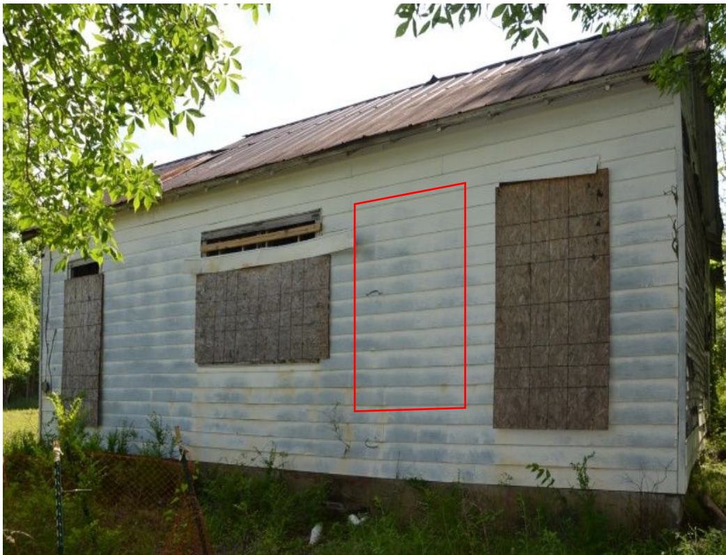
Image 7. One window from the 1927 classroom has been covered over entirely with new siding. Missing window represented by red box. Photo by Grace Abernethy.
