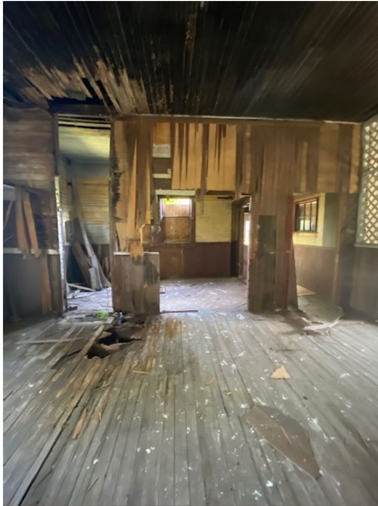
Image 11. Floorboards in current condition in the 1927 classroom. Photo by Rachael Finch.
