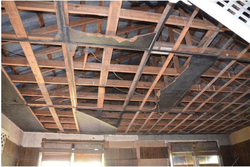
Image 14 (left). Walls and ceiling in the 1940s classroom. Photo by Grace Abernethy.
