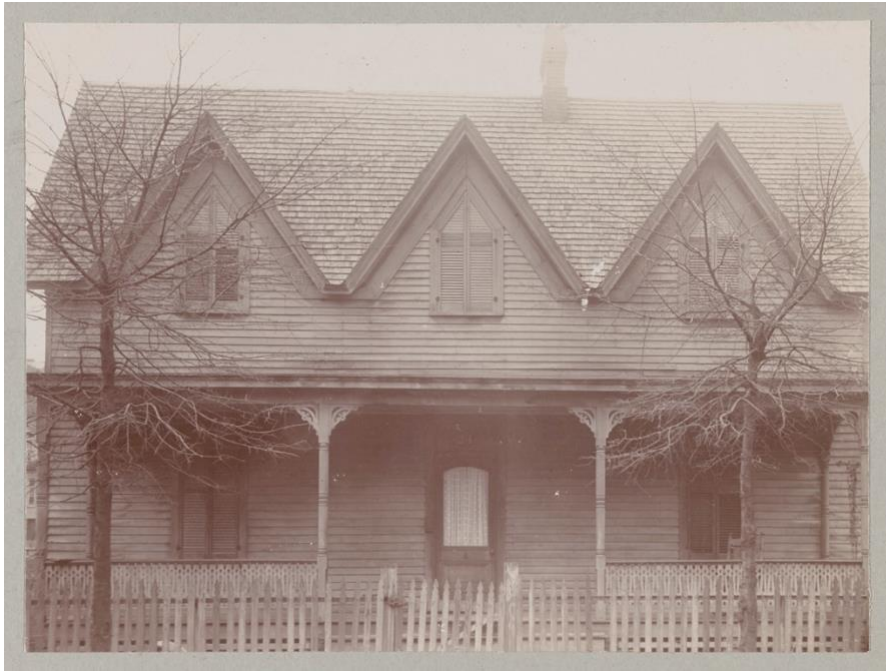
Figure 7: Home of N.E. Singleton, Chattanooga, Tennessee (1900). Photo courtesy of the Library of Congress.
