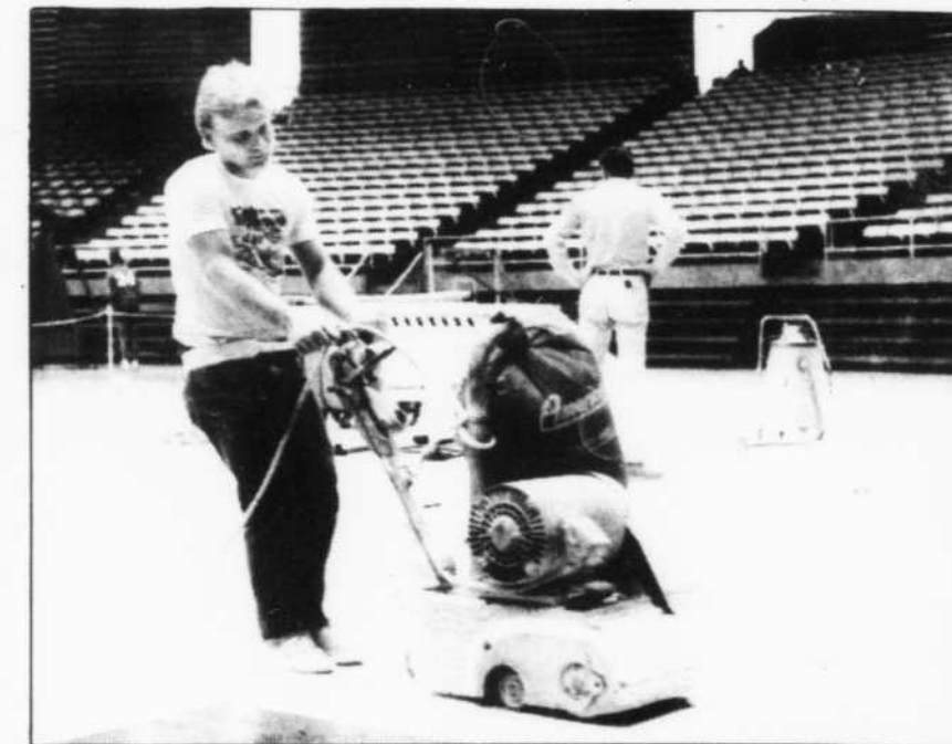
Terry Warrick, of Fyke Flooring Co., strips the finish off of the Murphy Center floor after last Tuesday's water damages.
