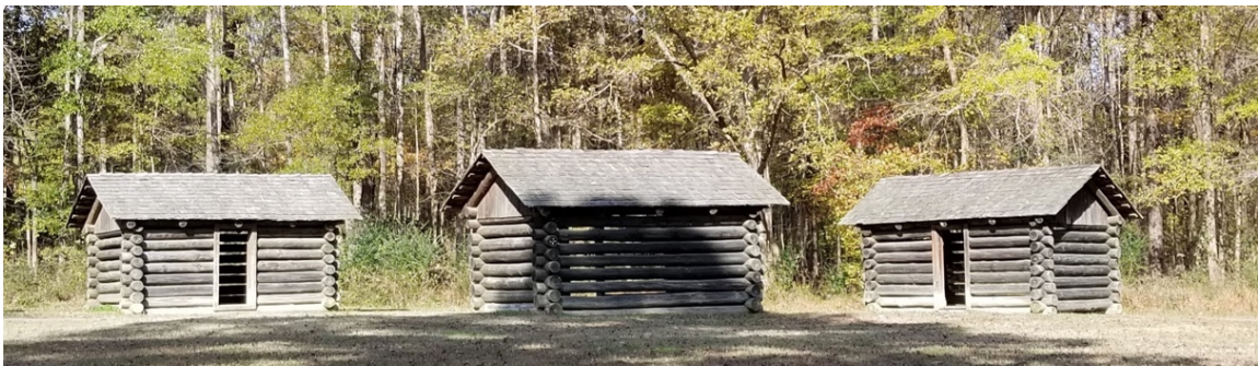
Figure 6-8. Reconstructed cabins built according to Featherstonhaugh's description. Courtesy of the author.
