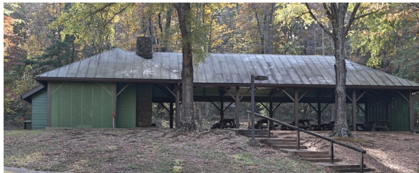
Figure 6-13. Picnic shelter. Courtesy of the author.
