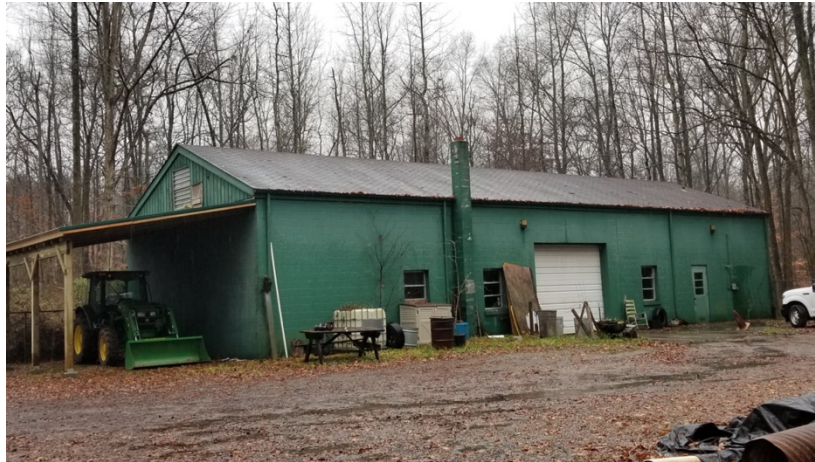
Figure 6-24. Maintenance building. Courtesy of the author.
