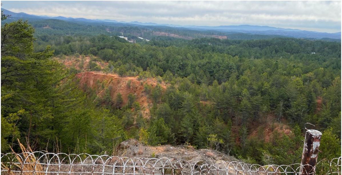
Figure 4. A collapsed mine in Ducktown, TN. (Ryan Barnes 01/03/2024)
