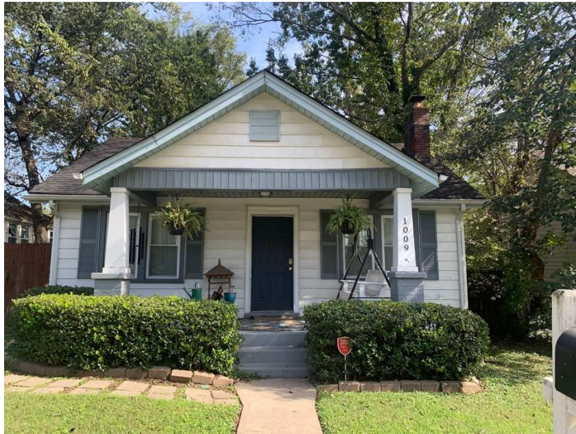
(Figure 2.11) 1009 North 6 th Street.
