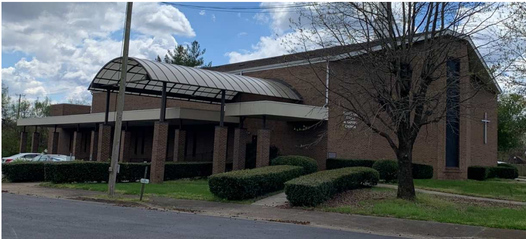
(Figure 2.36) 608 Cleveland Street, front view.
