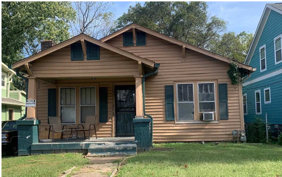
(Figure 2.13) 1213 North 6 th Street.
