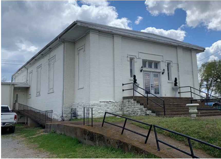
(Figure 2.31) 1201 Joseph Avenue in present-day.
