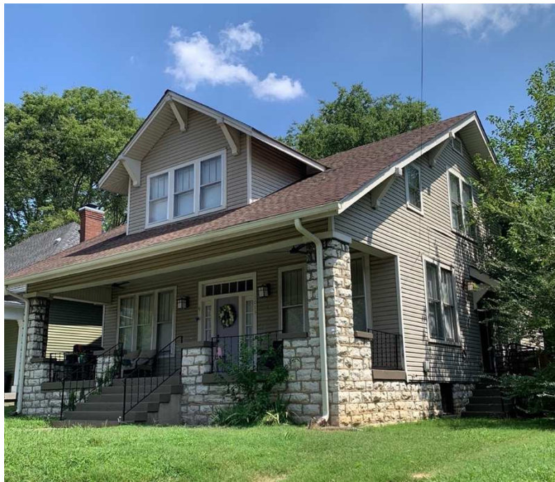
(Figure 2.9) 1013 North 5 th Street.
