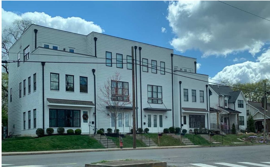
(Figure 2.22) 1225 North 5 th Street.
