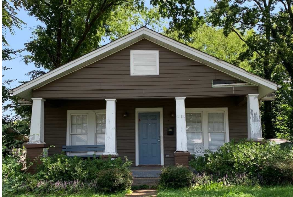
(Figure 2.12) 1115 North 5 th Street.
