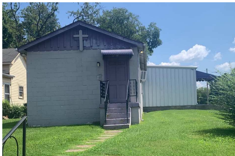
(Figure 2.39) 1005 North 5 th Street.
