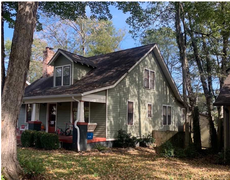
(Figure 2.10) 1111 North 6 th Street.
