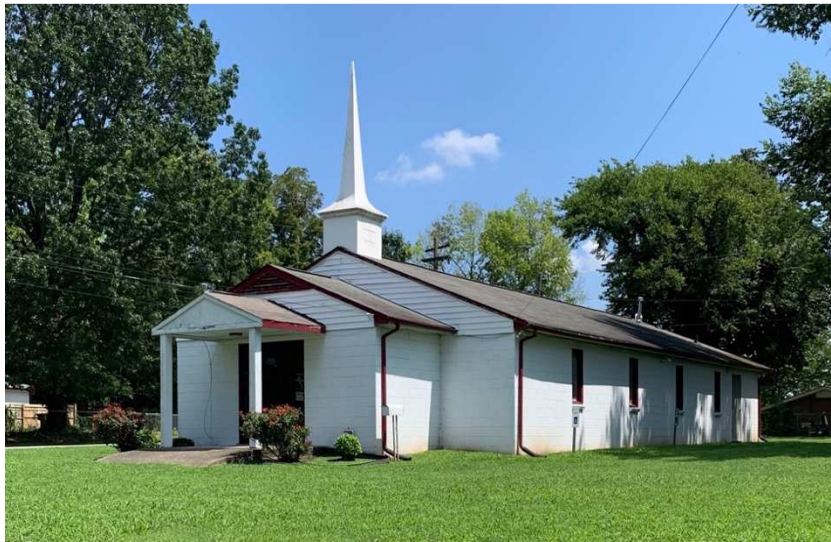
(Figure 2.38) 1027 North 5 th Street.
