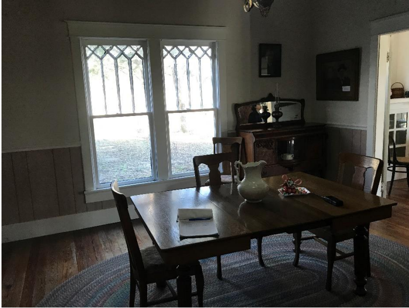
Figure 3.2. Image of original wood windows with diamond encasement design. Photograph taken by author, 2020.
