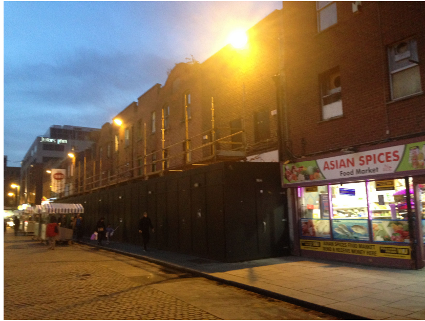
Fig. 15. Moore St. no. 14-17, the fronts covered in scaffolding. (photo by Author)
