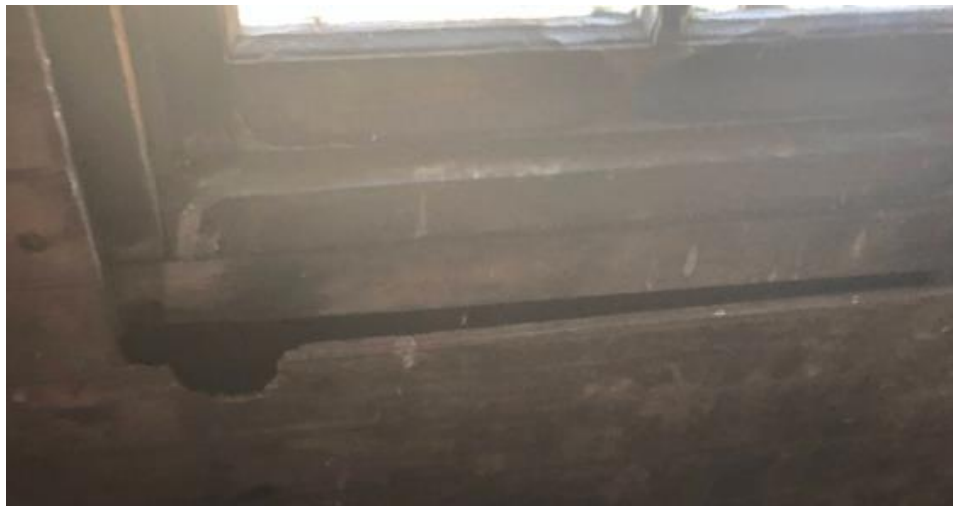
Figure 31. Gap under window in the west second-floor bedroom on the west wall. Photo provided by Abigail Coomes.
