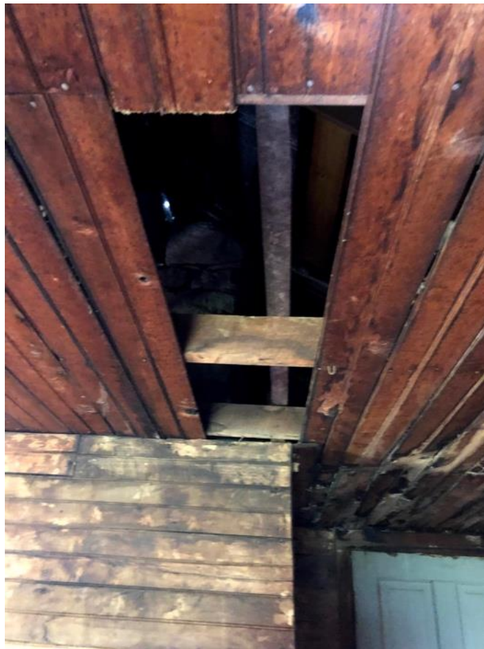
Figure 33. Missing panels in the ceiling of the west second-floor bedroom. Photo provided by Abigail Coomes.
