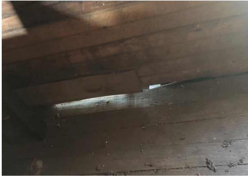
Figure 32. Gap under the north wall in the west second-floor bedroom. Photo provided by Abigail Coomes.
