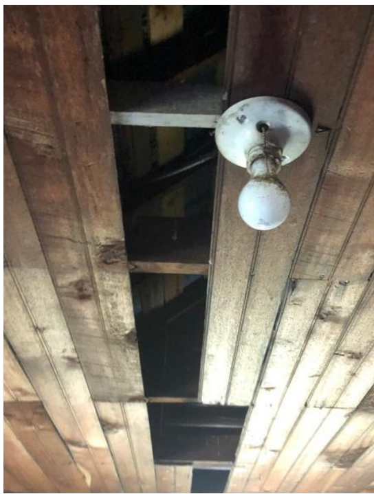
Figure 34. Missing panels in the ceiling of the east second-floor bedroom. Photo provided by Abigail Coomes.
