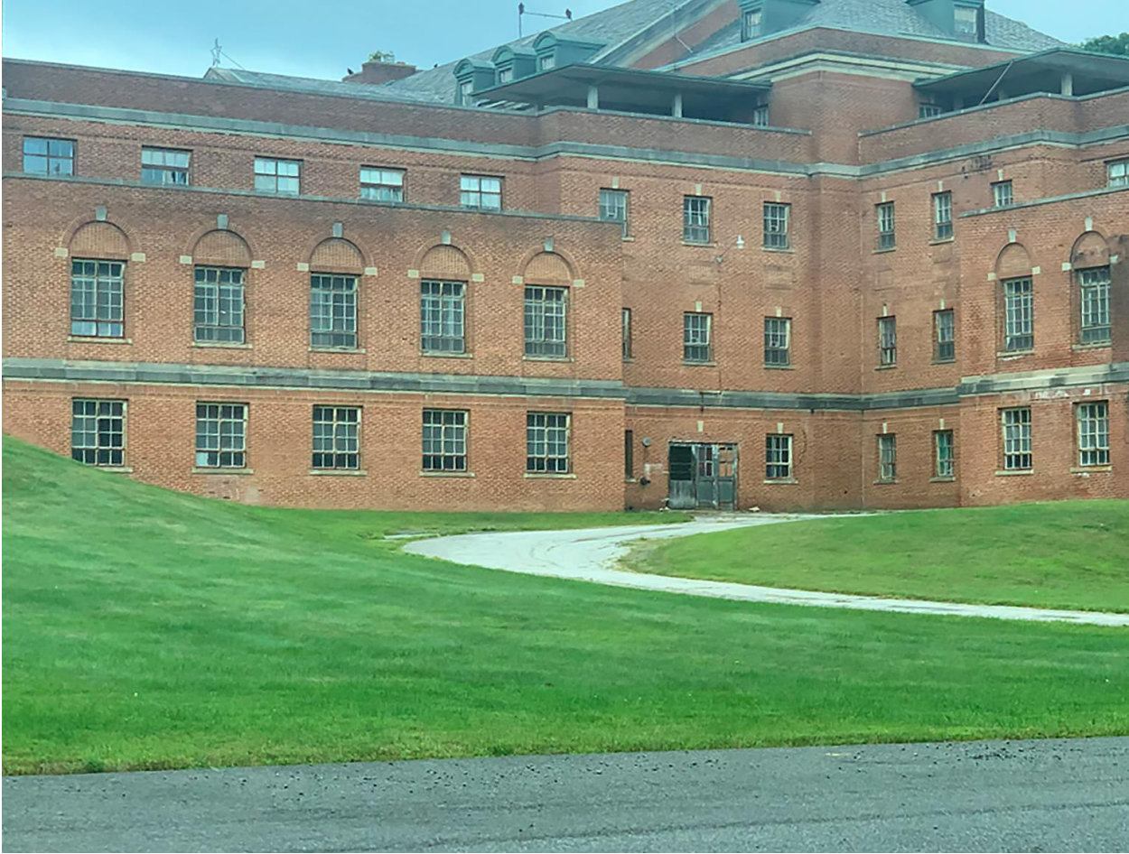
Figure 37. Rear of Preventorium
