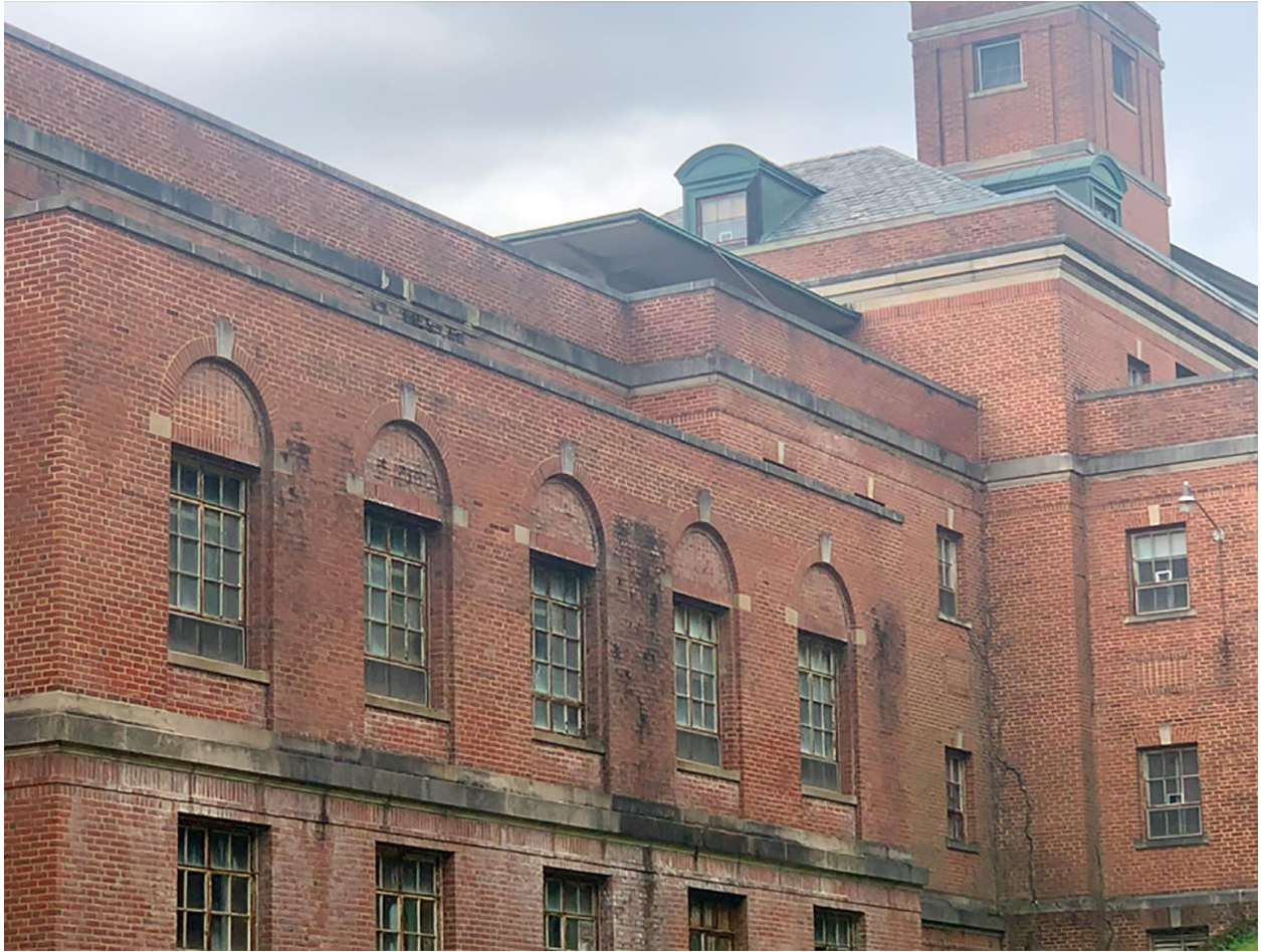
Figure 35. Preventorium sleep porch in distance
