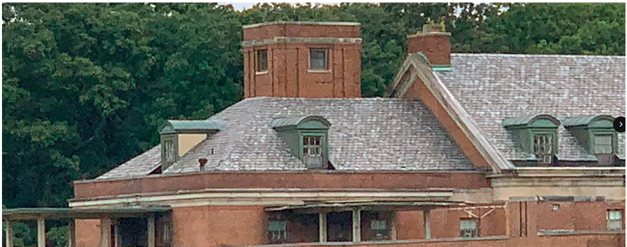
Figure 91. More gable-roofed windows of preventorium
