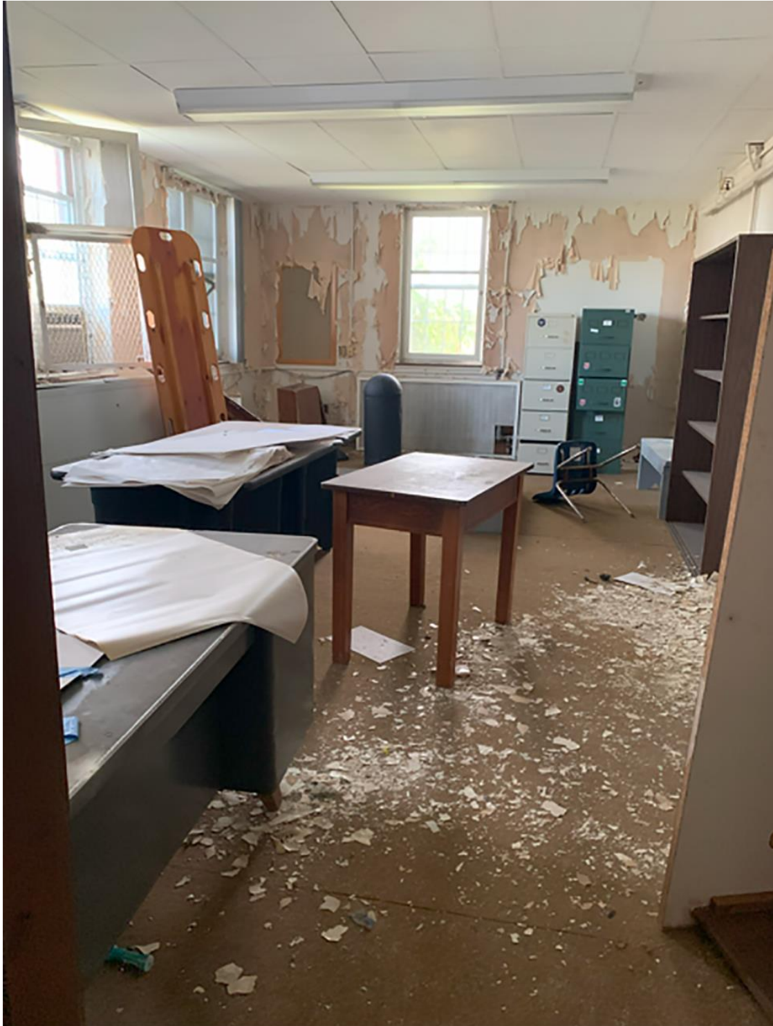
Figure 18. Interior of former patient room - changed to storage space for prison
