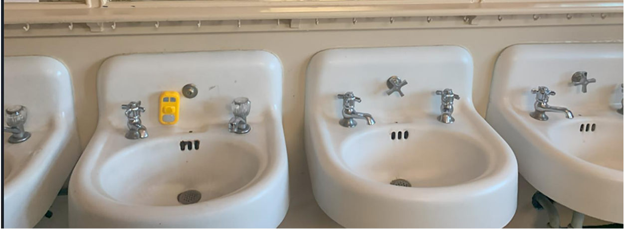
Figure 54. Original children's sinks
