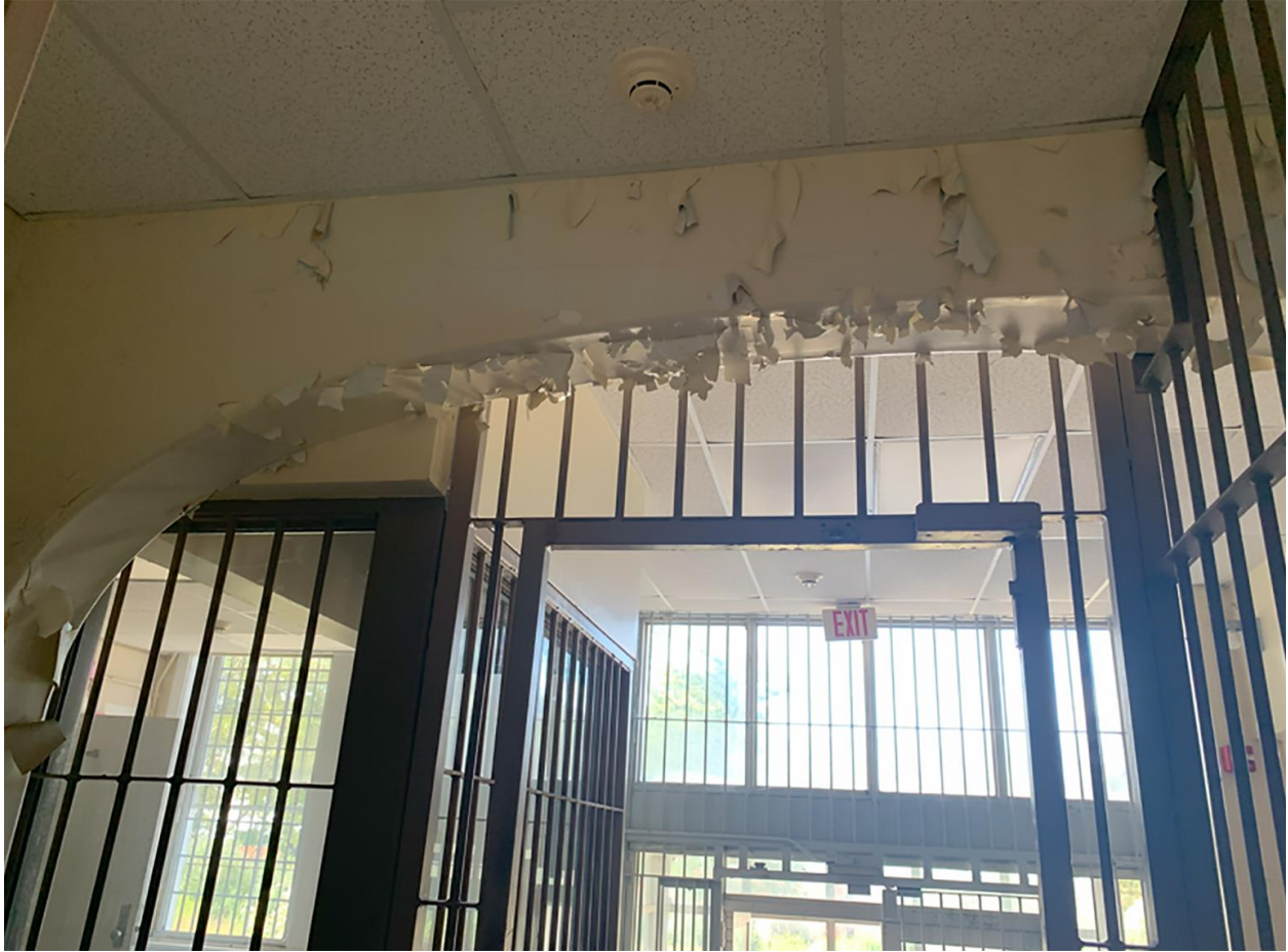
Figure 26. Detail of prison renovation of historic building
