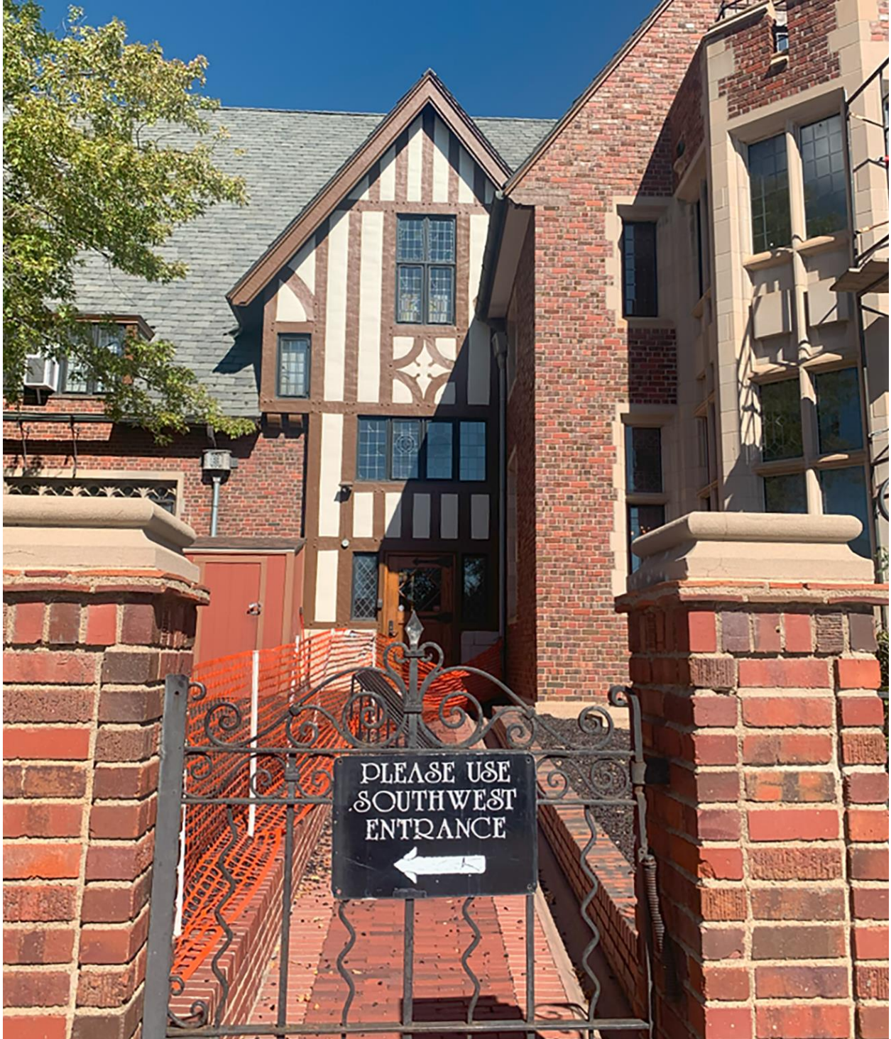
Figure 48. Front entrance of daycare
