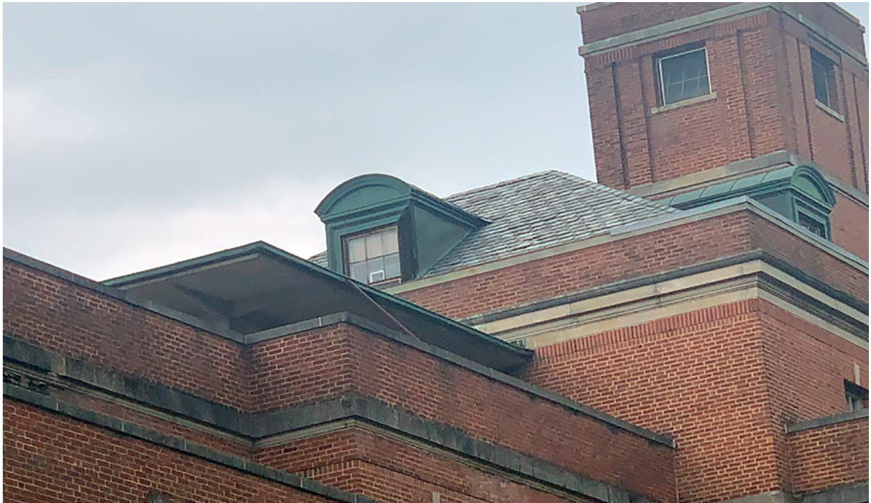
Figure 90. Gabled roofed windows of preventorium
