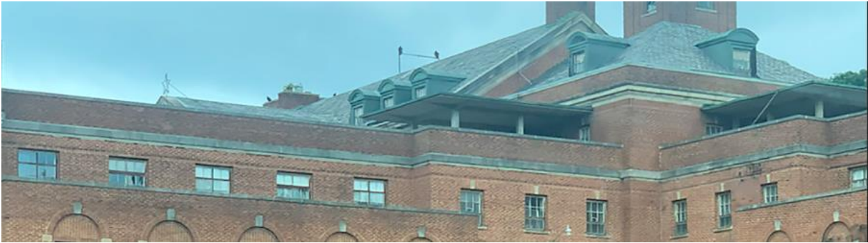
Figure 57. Close up of preventorium sleeping porch
