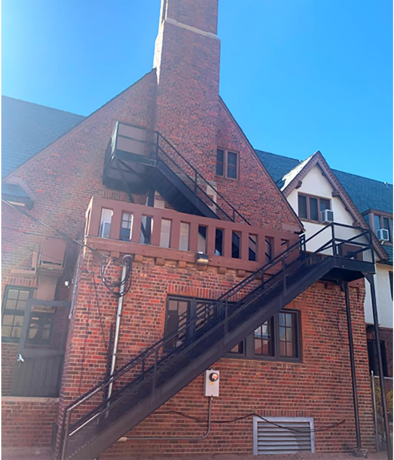
Figure 50. Rear of Daycare
