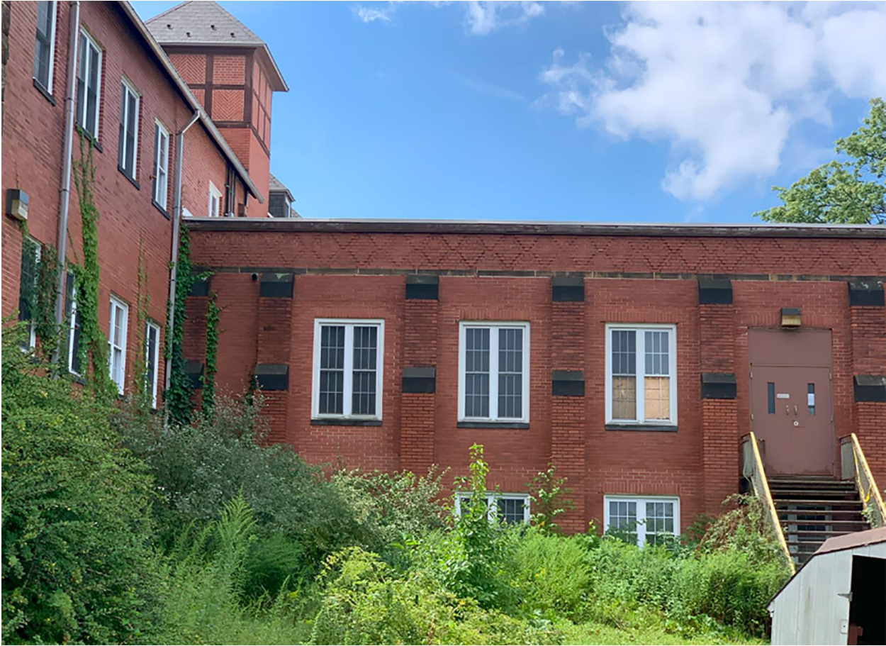
Figure 13. Close up of Maple House behind
