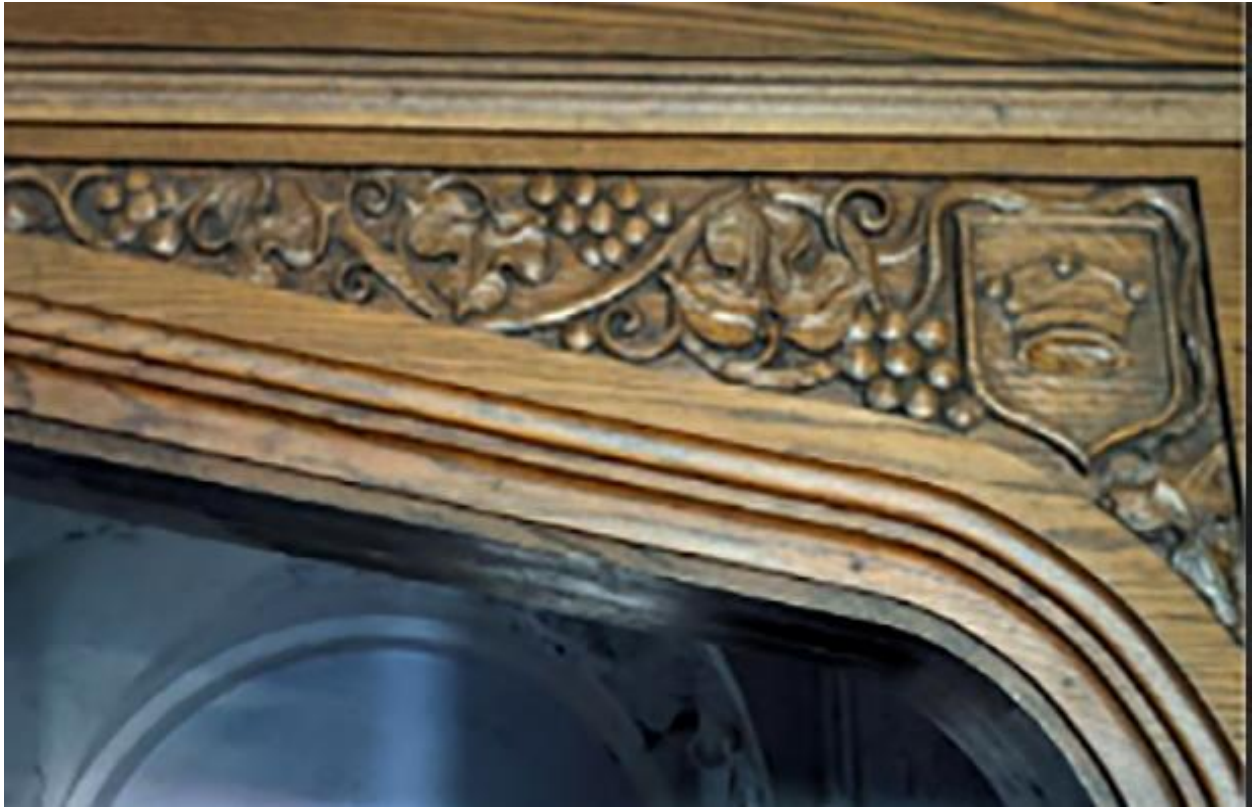
Figure 79. Detail of Maple House door
