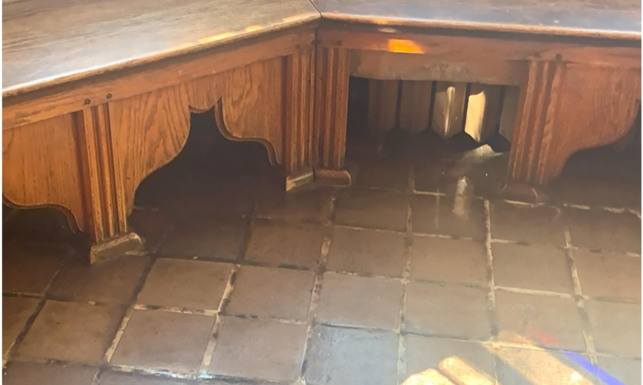
Figure 118. Scalloped detailing of original children's benches
