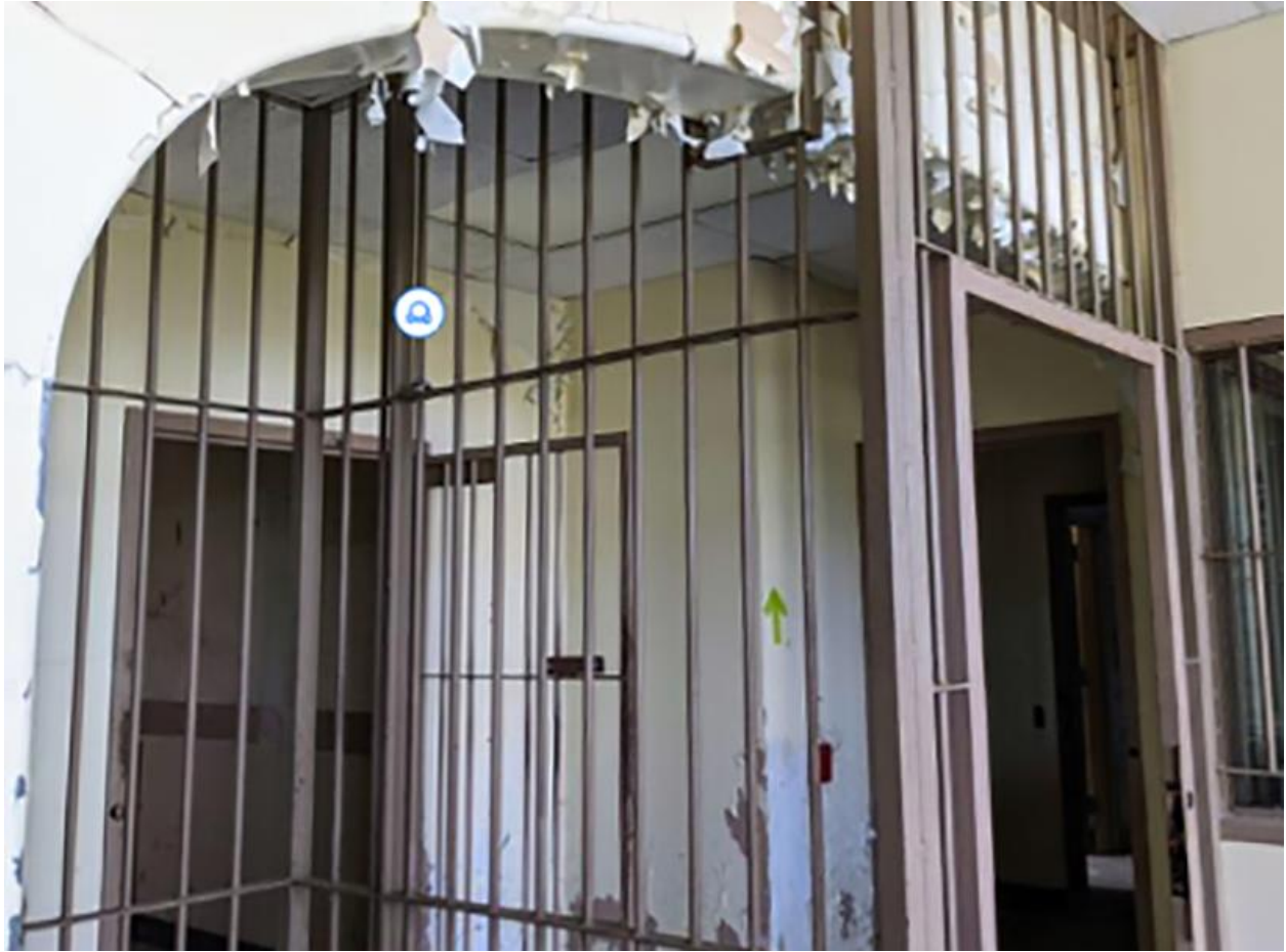
Figure 25. Example of prison renovations to original administration building
