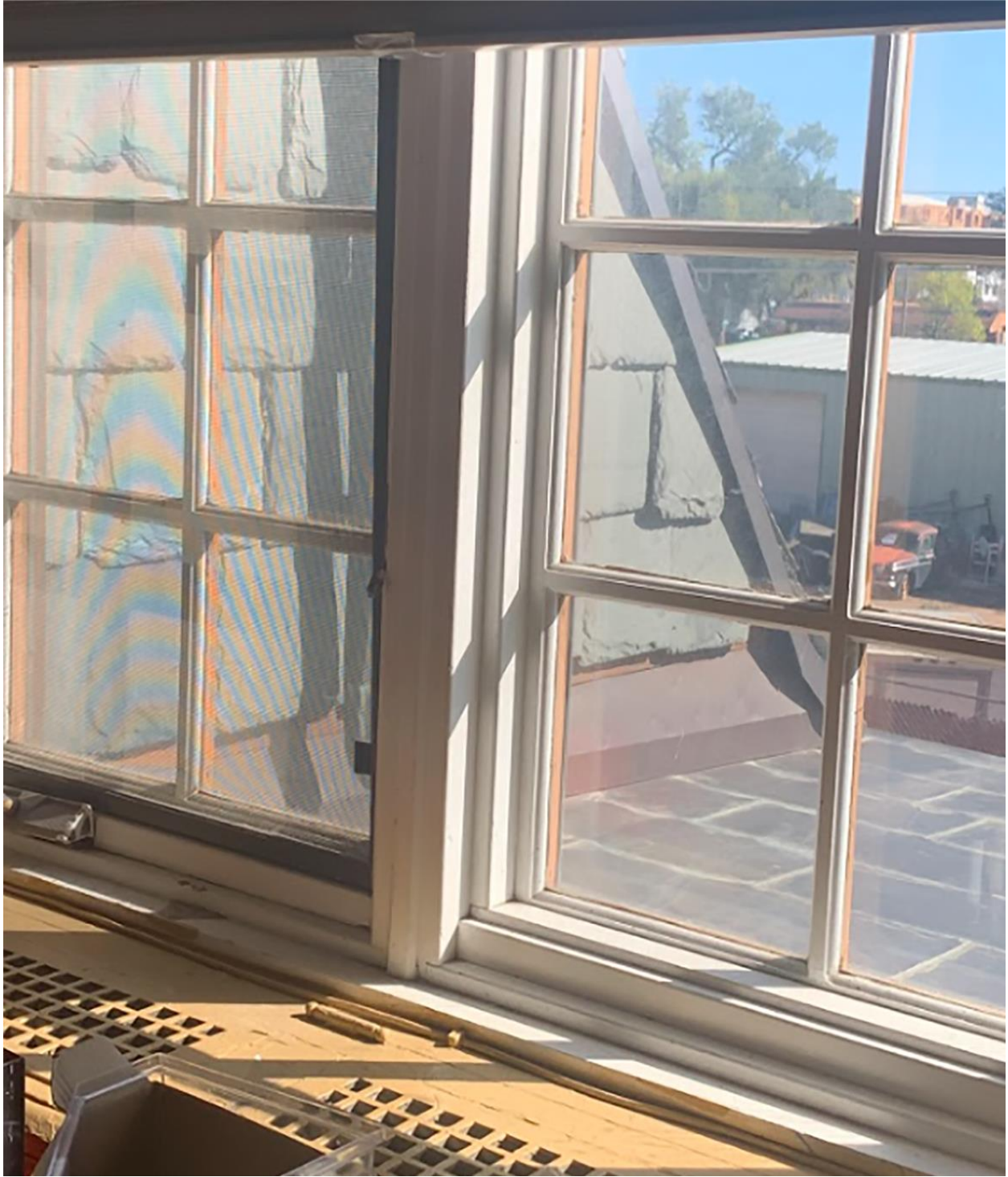
Figure 60. Partial side view of sleeping porch through window
