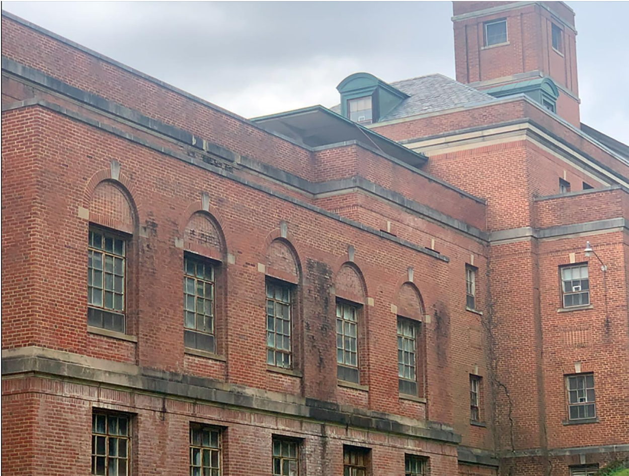
Figure 56. Rear of Preventorium - sleeping porch in distance
