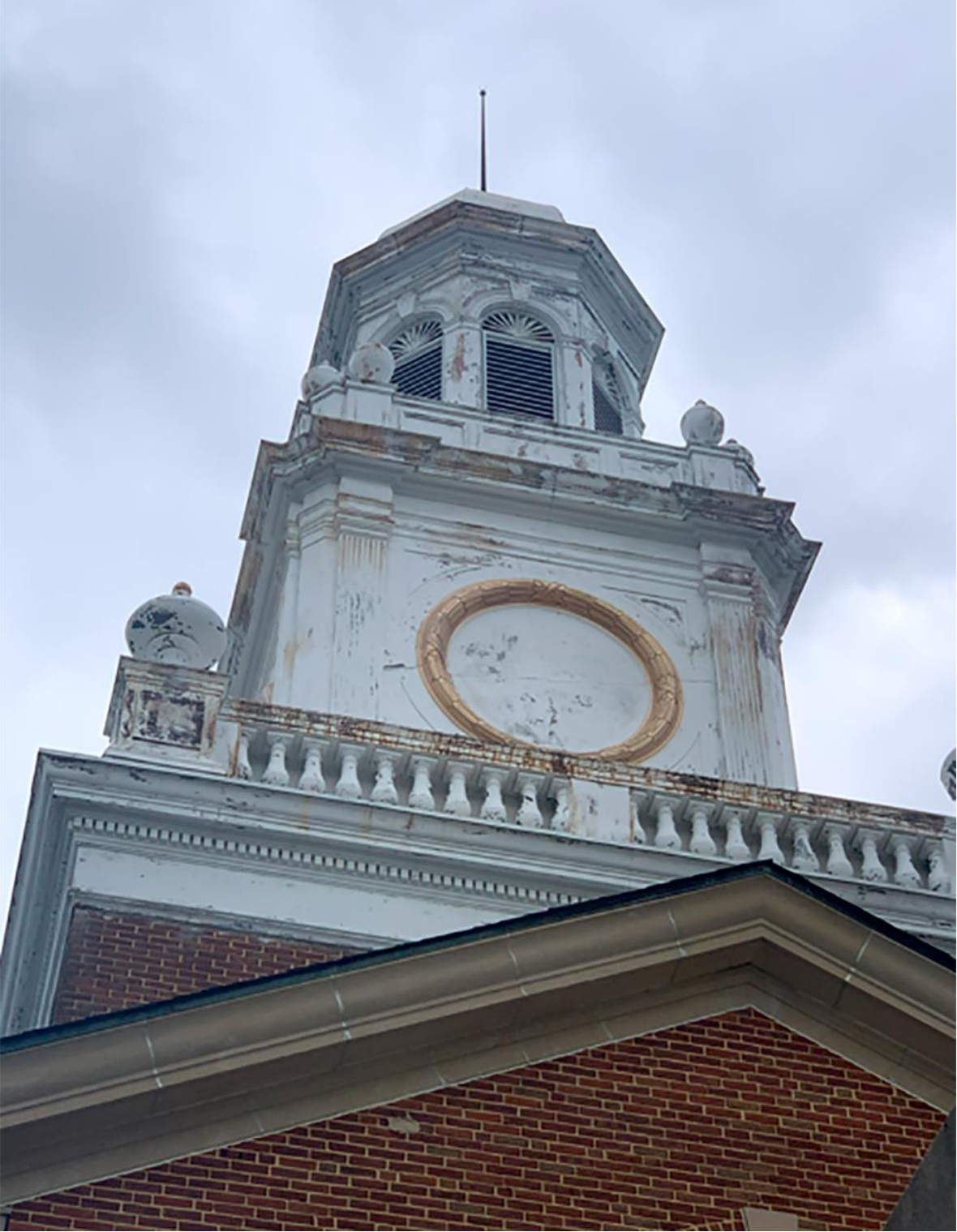
Figure 97. Copula on administration building
