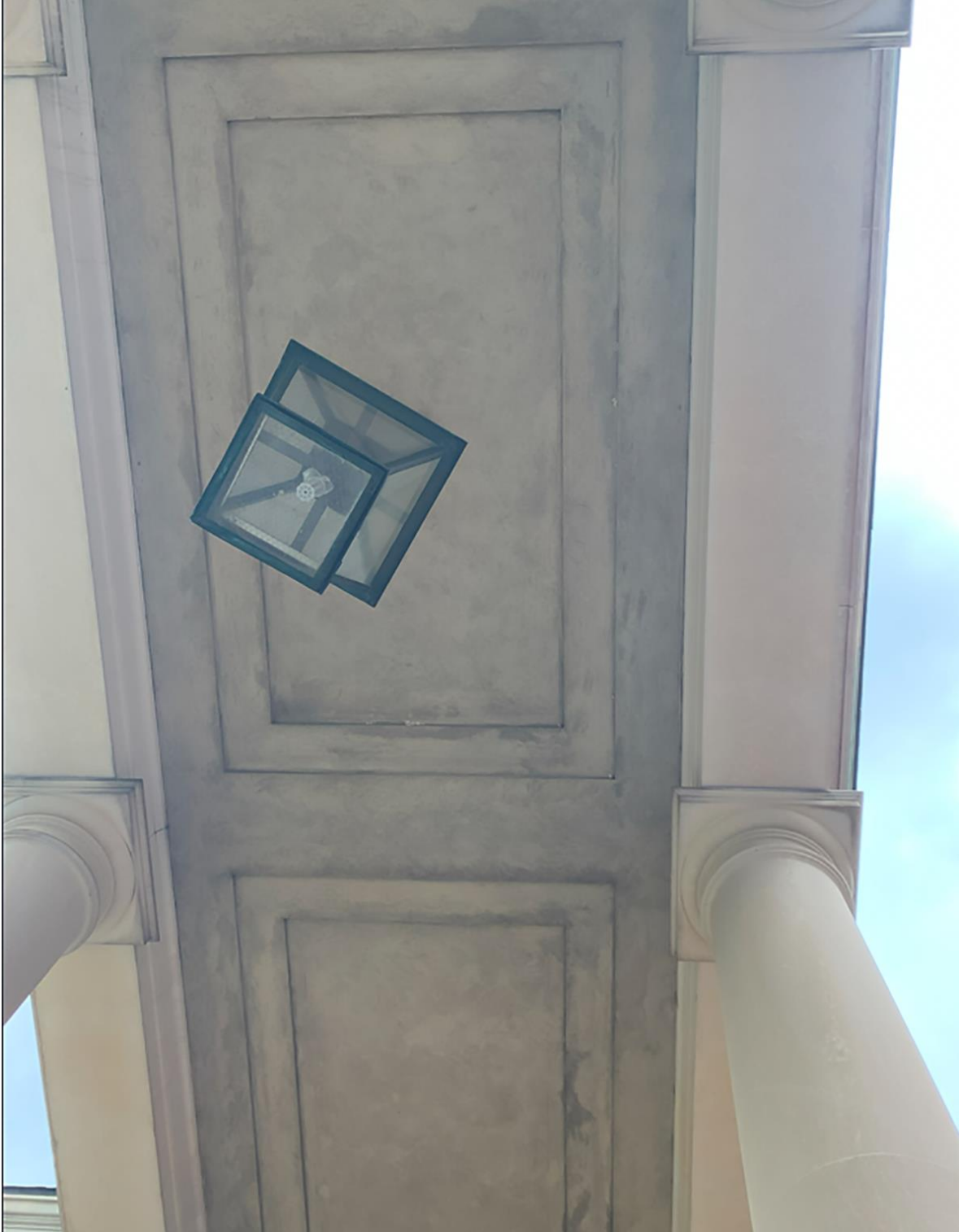
Figure 99. Ceiling of Sleeping Porch
