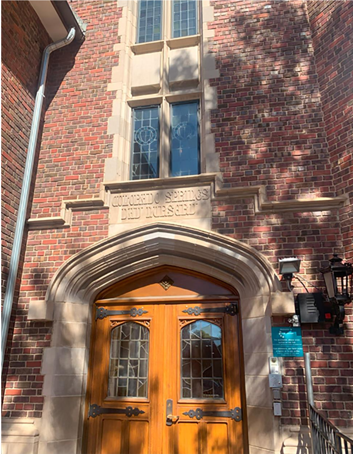
Figure 104. Decorative trim of door and view of stained glass
