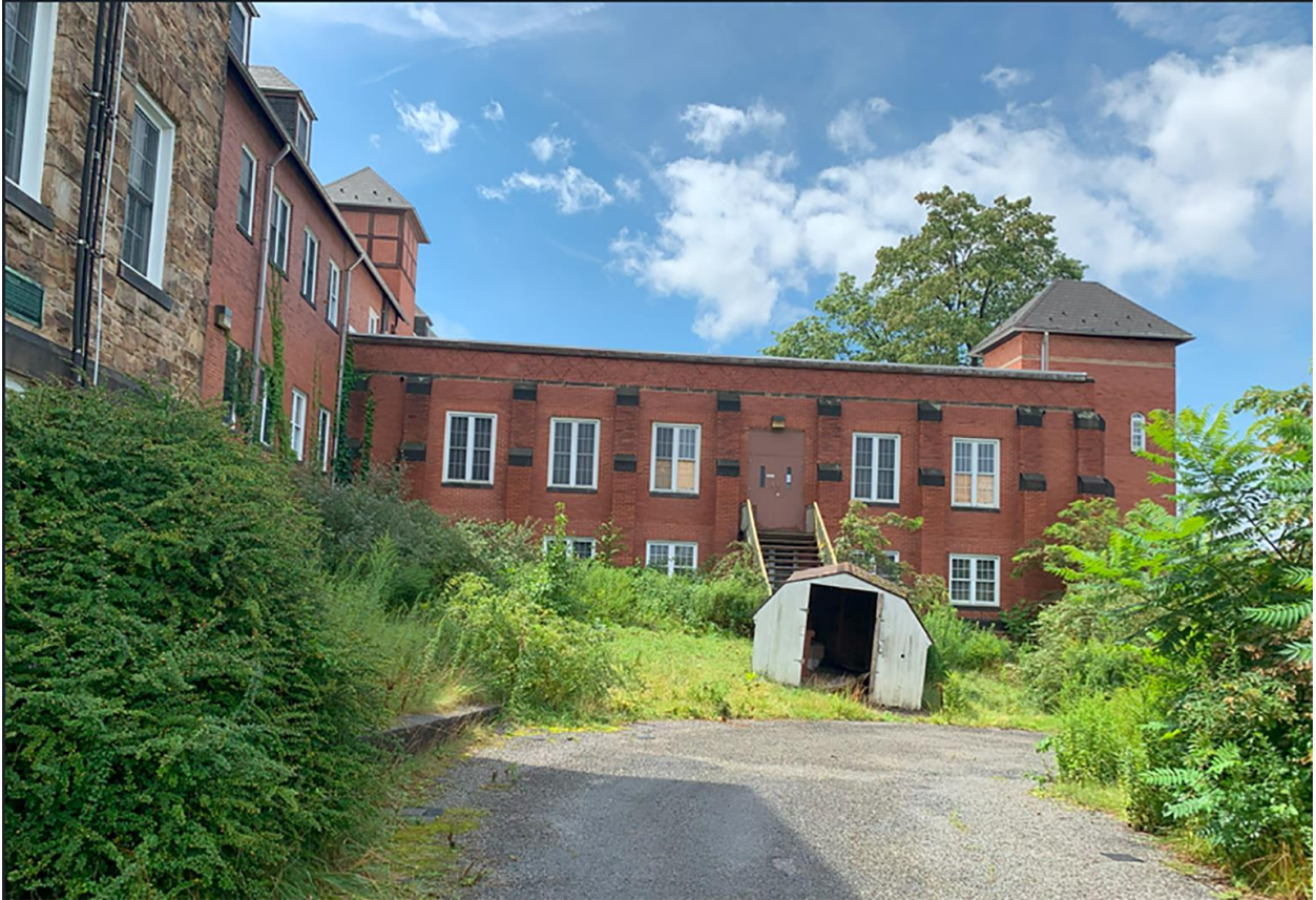
Figure 12. Back of part of Maple House
