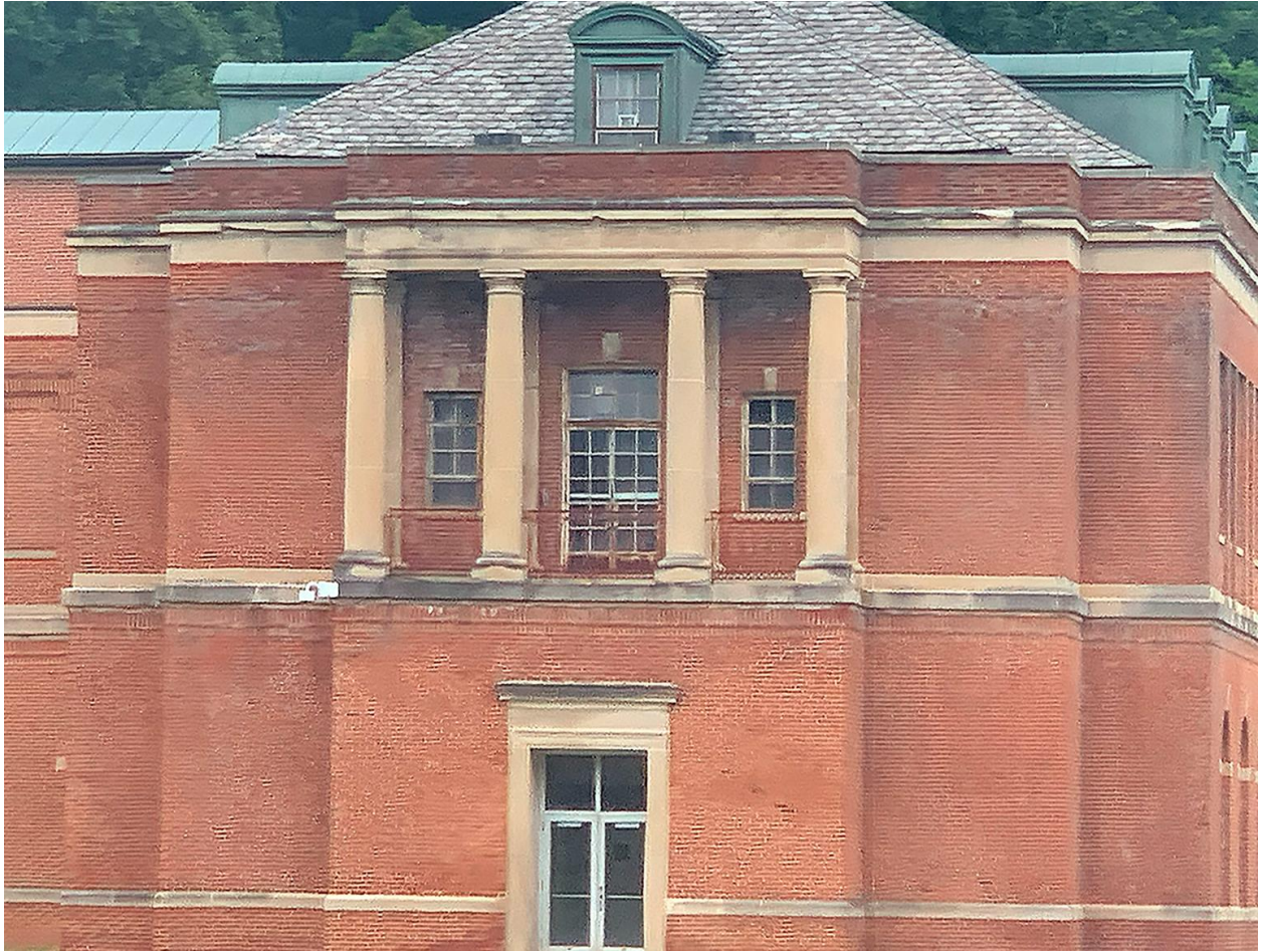
Figure 38. Rear of preventorium - close up of columns
