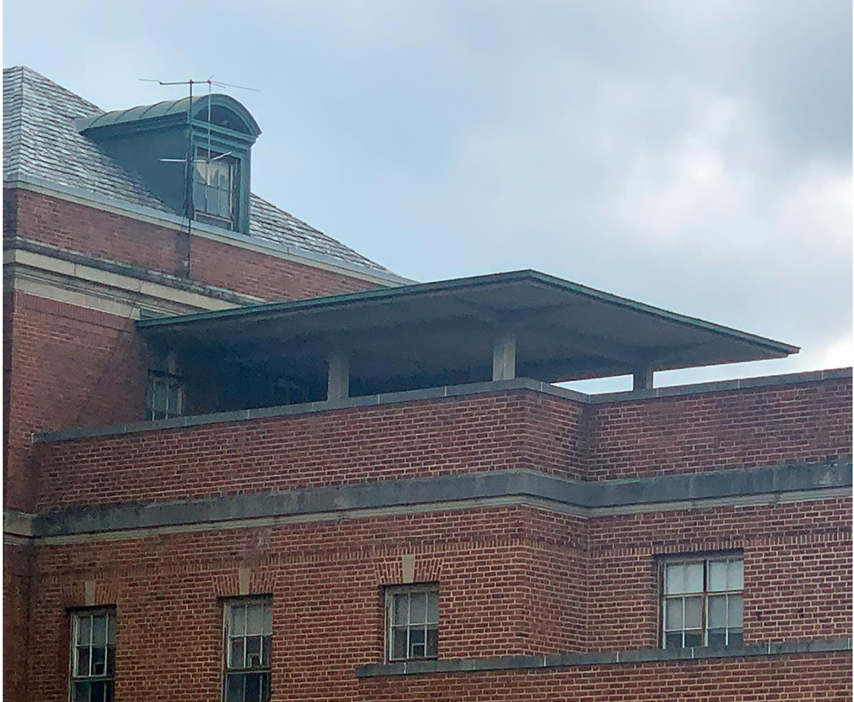
Figure 58. Close up of preventorium sleeping porch
