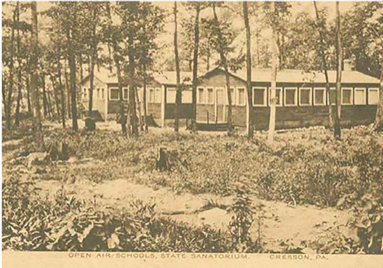
Figure 65. Cresson open-air school
