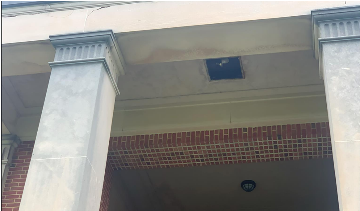
Figure 96. Column frieze and brick trimming
