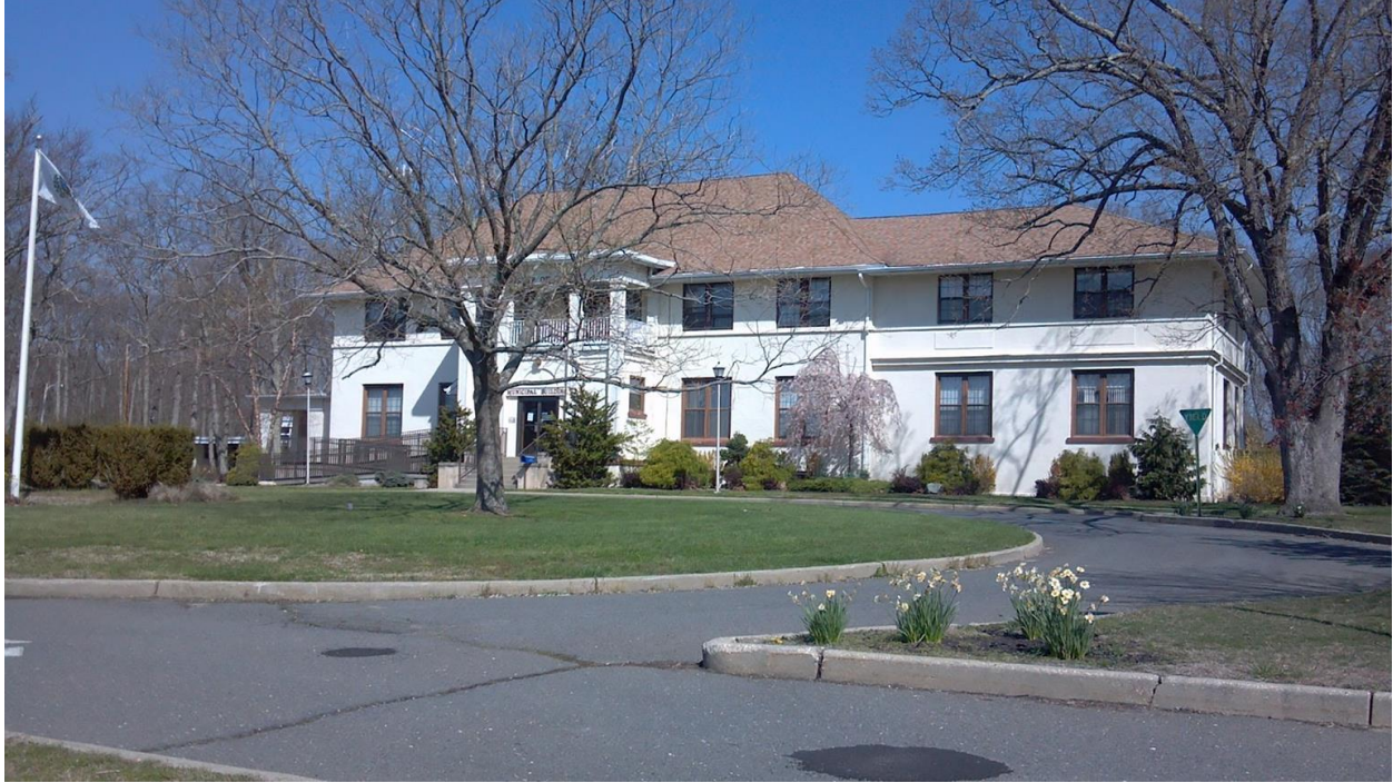
Figure 2. Distant view of Town Hall
