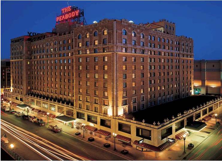
Figure 5.1: The Peabody, Exterior, in Memphis Tennessee (2016)
