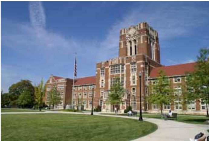
Ayres Hall on UT-Knoxville campus
