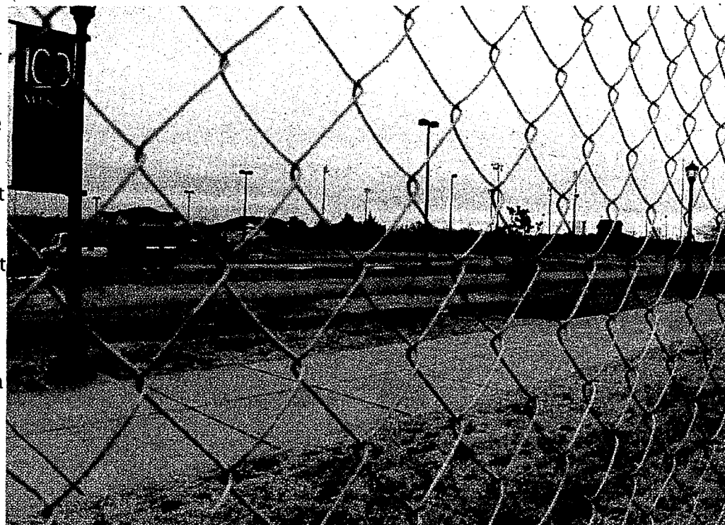
The Rec Center lot, formerly used by students, lies vacant as construction for the new parking garage is slated for Jan. 27, according to Malone. Photos by Kelsey Klingemeyer, photo editor
