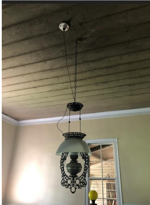
Dining room light fixture retrofitted with modern bulb. Photo taken by CHP Staff.
