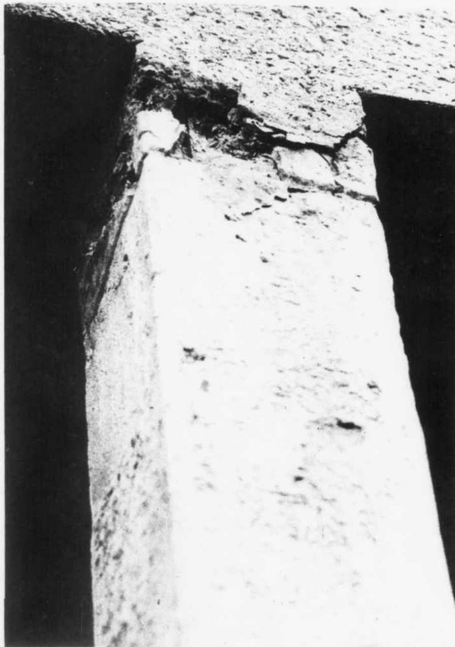
U.C. columns await warmer weather for repair.
