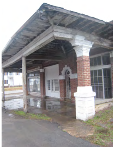
Abston Garage, Oliver Springs
