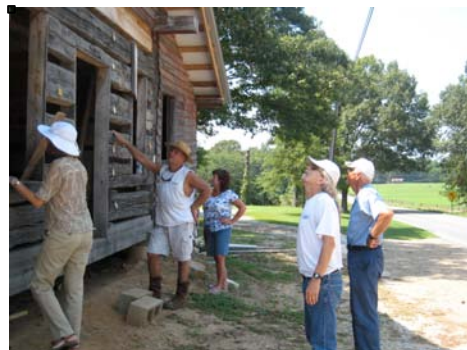
Heritage Area's preservation specialist Michael Gavin advises on the restoration of Dunbar's Keeton Store (Decatur Co).
