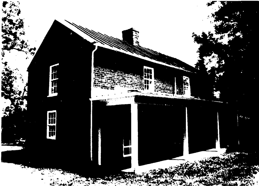
Fig. 2-3. Southern tenant house.
