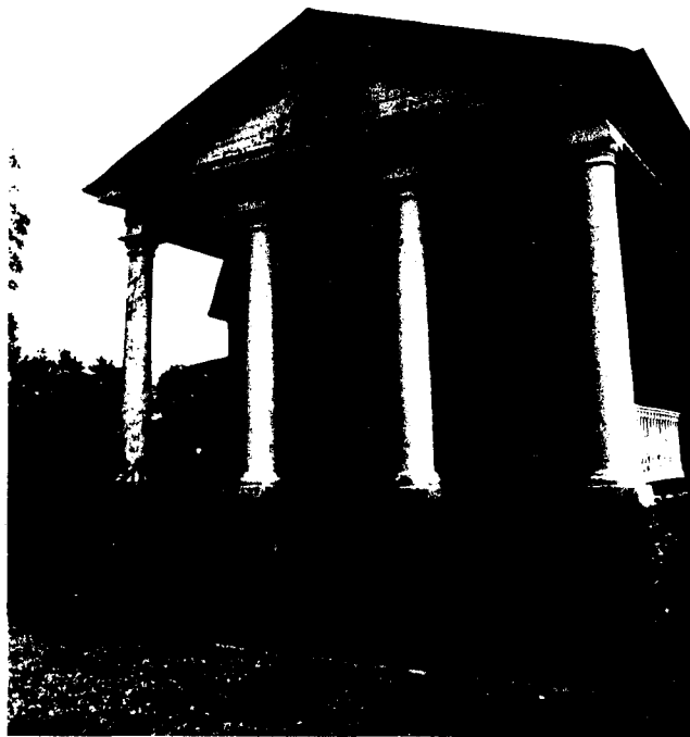
Fig. 3-6. Detail of classical portico on front facade.
