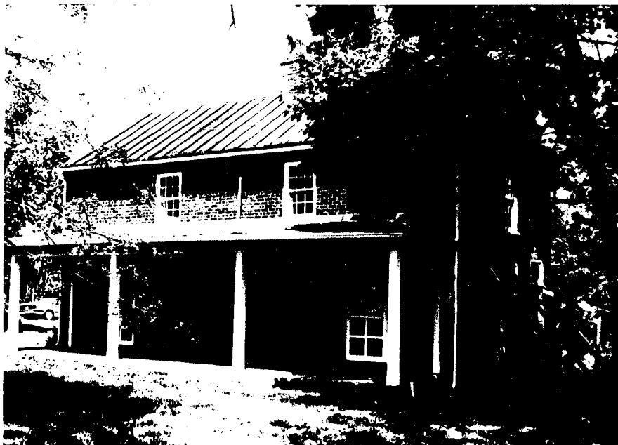
Fig. 5-1. Southern tenant house.
