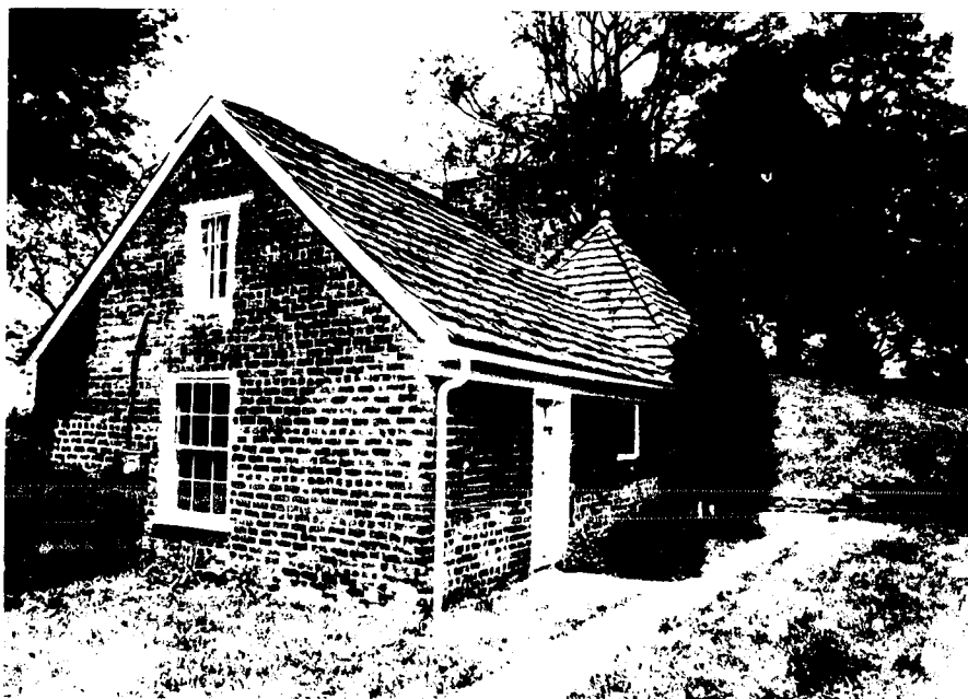
Fig. 5-3. Remaining kitchen and smokehouse.
