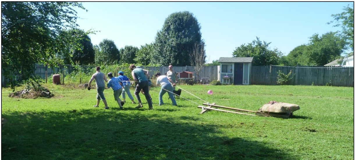
Figure 6 Construction Team Moving the First Stone with a Sled
