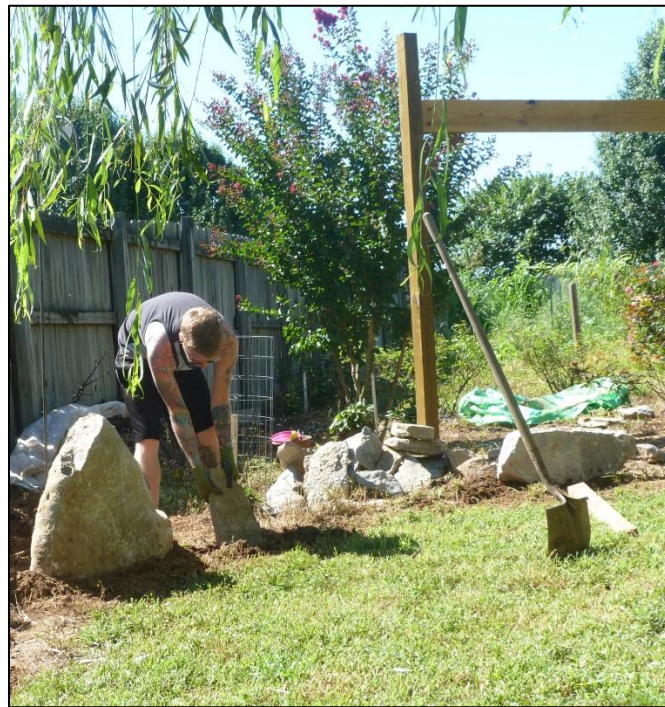
Figure 8 Setting the Perimeter Stones
